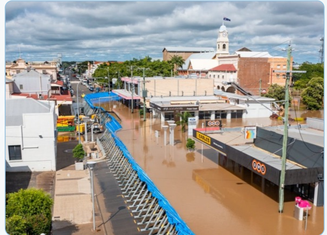
Fast-deploying flood barriers installed in Maryborough Queensland, March 2022
