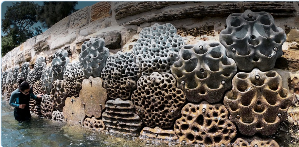
Biodiversity-enhancing elements added to a protective seawall in Sydney, Australia, courtesy LivingSeaWalls .
